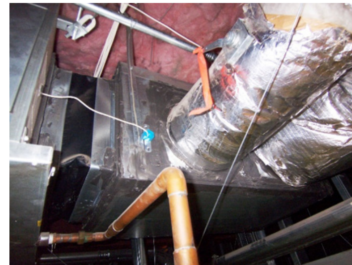
TYPICAL FAN COIL UNIT
