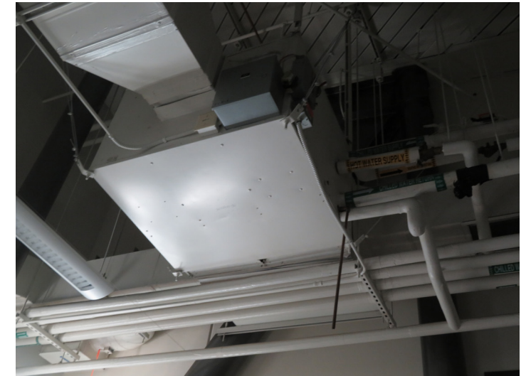
TYPICAL FAN COIL UNIT
