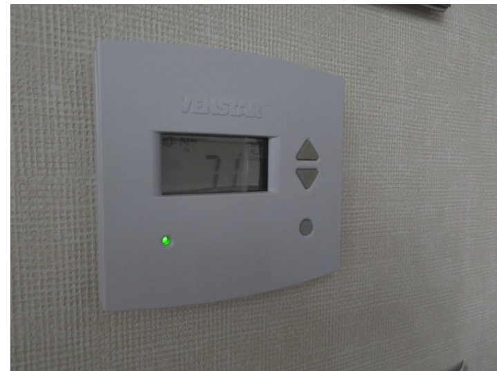
TYPICAL PROGRAMMABLE THERMOSTAT
