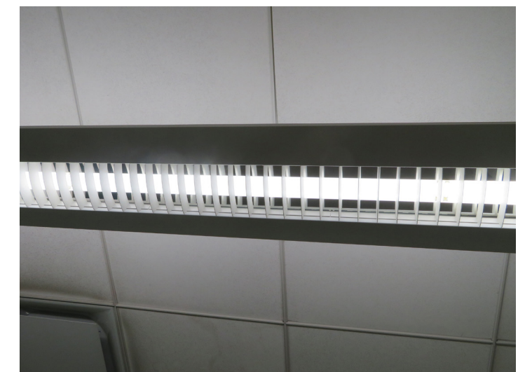
TYPICAL CLASSROOM FIXTURE WITH F32T8 LAMP
