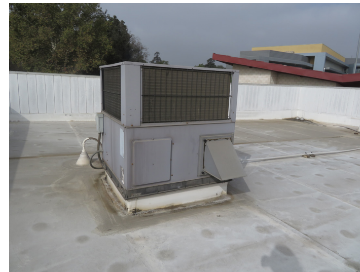
TYPICAL PACKAGED ROOFTOP HEAT PUMP
