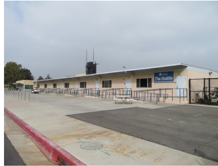
COMPUTER TECHNOLOGY SERVICES BUILDING
