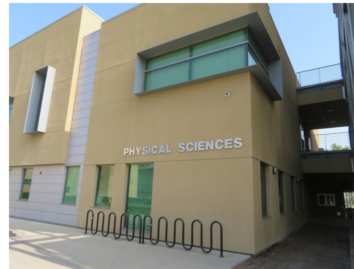
PHYSICAL SCIENCES BUILDING
