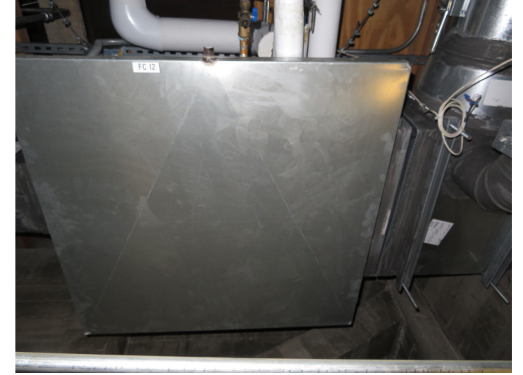
TYPICAL FAN COIL UNIT
