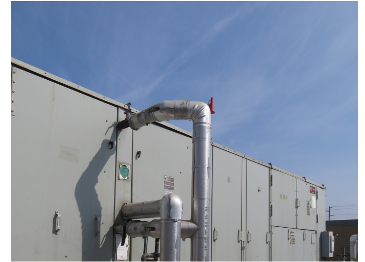
TYPICAL AIR HANDLER WITH CHILLED WATER CONNECTION
