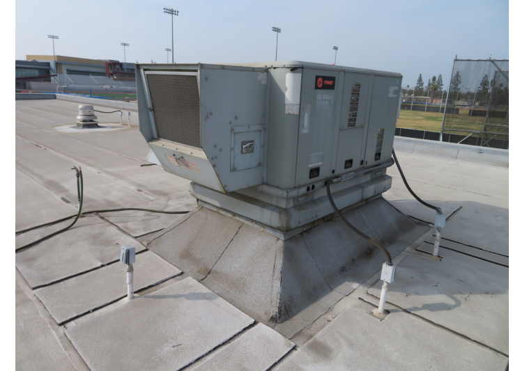
TYPICAL PACKAGED ROOFTOP HEAT PUMP
