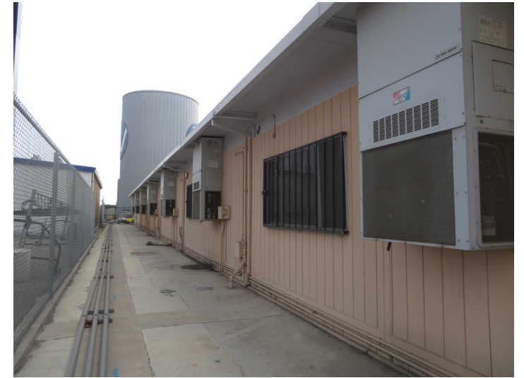
WALL-MOUNTED HEAT PUMPS
