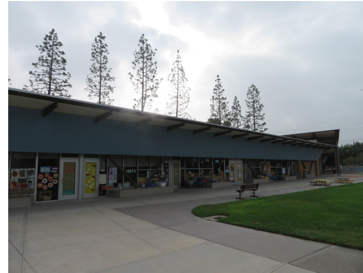
CHILD DEVELOPMENT CENTER CLASSROOM BUILDINGS
