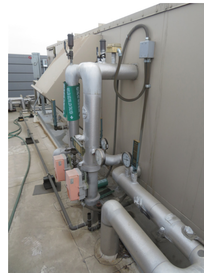
CHILLED WATER CONNECTION TO AIR
