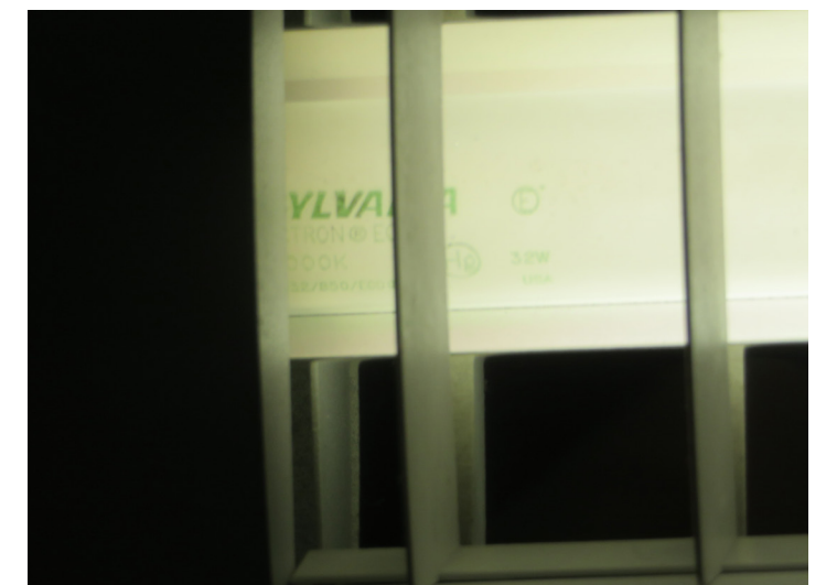
TYPICAL LIGHTING FIXTURE WITH F32T8 LAMP
