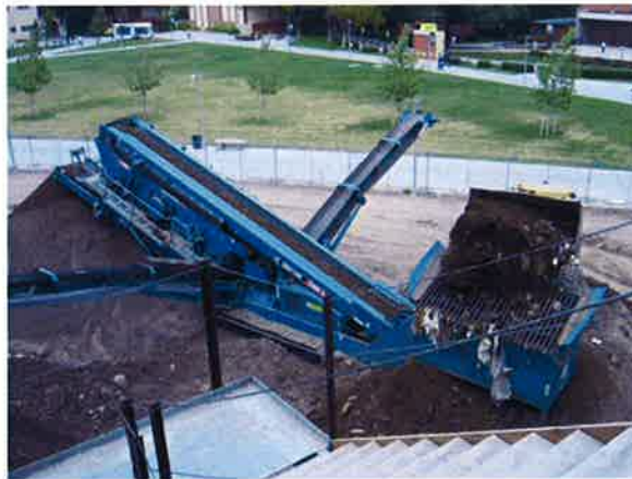
Screening soil for backfill
