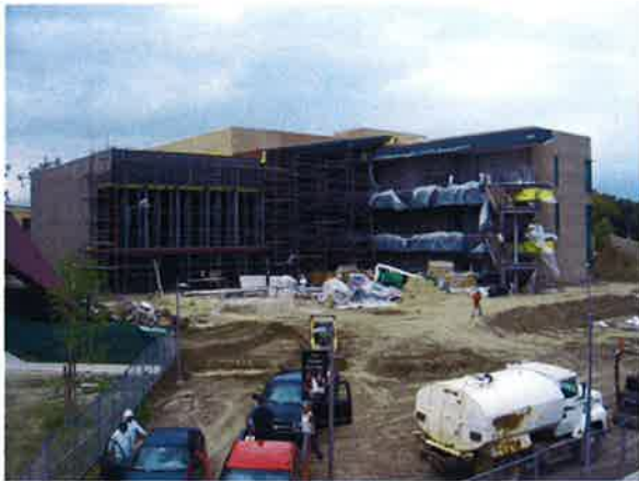
View from Business Building
