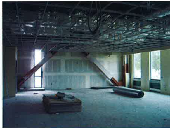
Ceiling grid installed
