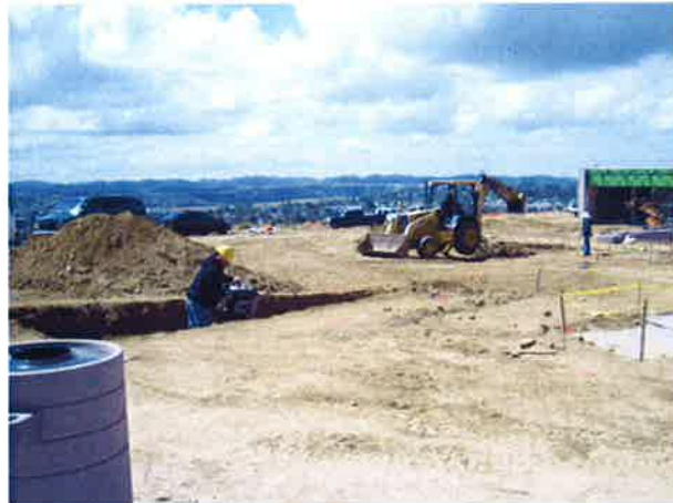
Grading for walkways and planters
