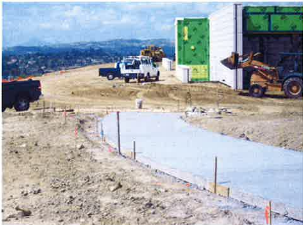
Concrete is being placed on walkways to LRC
