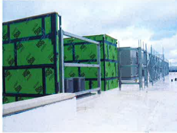
Rooftop HVAC Protection Installation
