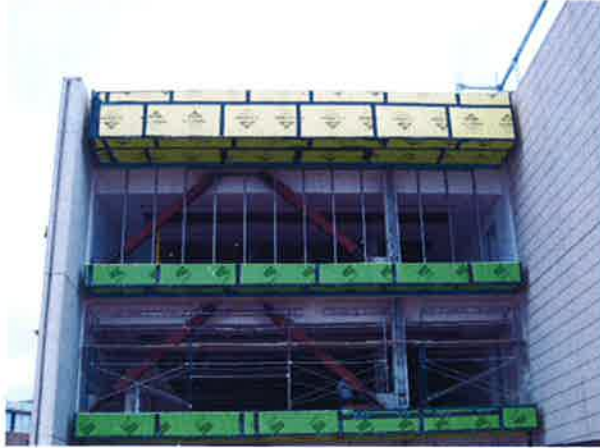
Beginning of wall curtain Installation
