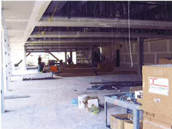
Progress on Upper level of Library
