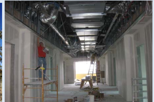
Work Progress at Lab Wing Building
