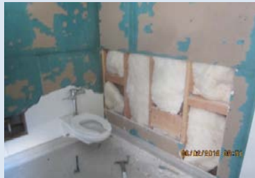
Modular Restroom Upgrades
