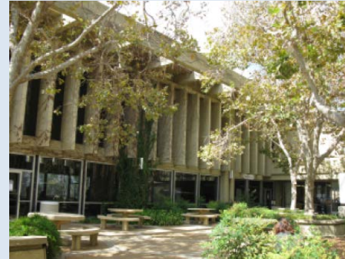
Exterior Building Photo of East elevation
