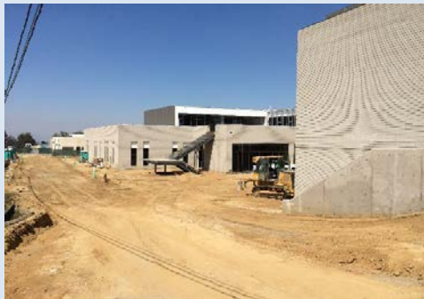
South Elevation With Metal Panels & CMU
