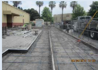
West Side Sidewalk work
