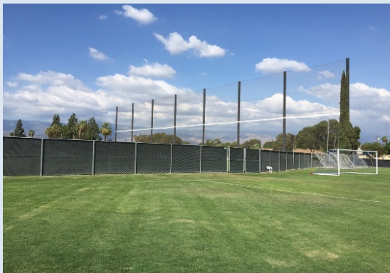
Future location for the netting fence
