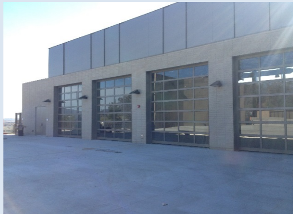
Fire Engine Bays
