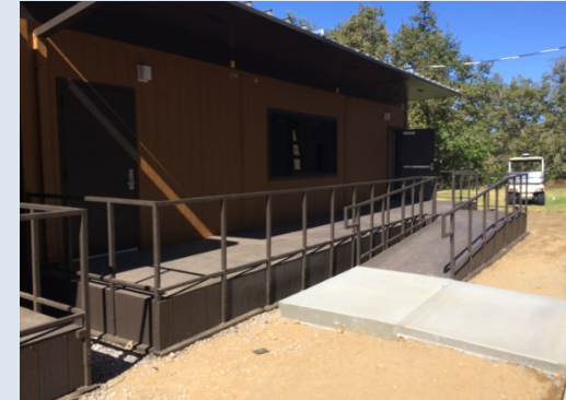
Modulars installation complete
