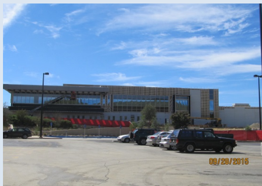
North elevation and partial Parking Lot C turn-over
