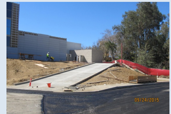
Ramp and asphalt base at Parking Lot C
