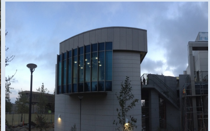
Work Progress at Lecture Wing Building
