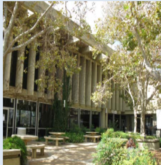
Exterior Building Photo of East elevation
