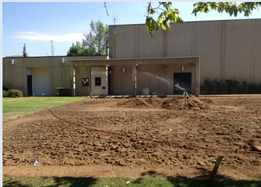
Grading of land for modular classrooms
