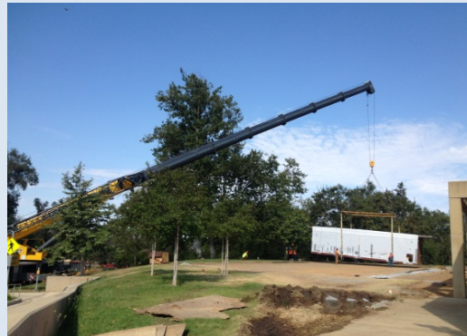
Modulars being installed next to the Gym
