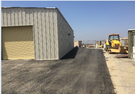
Exterior of New Warehouse
